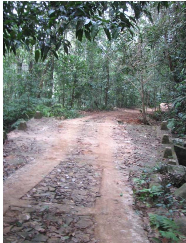
Photo 2: Concreted road and road widening in early 2000 (Photo: Prof IAUN Gunatilleke)
